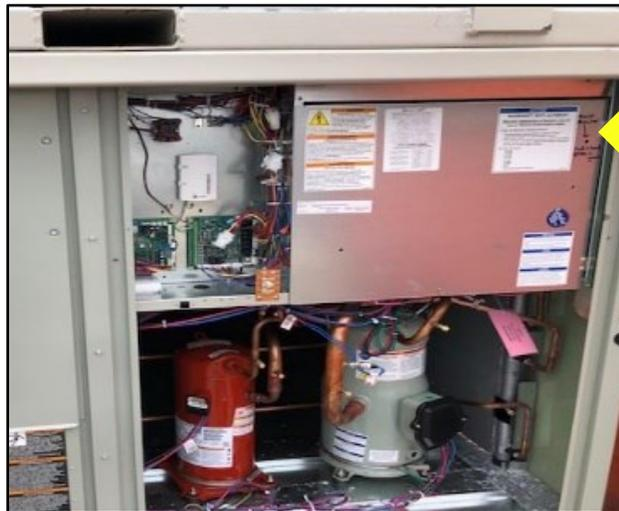
Remove outer door (right of unit) to expose Phase Monitor and Site Glass
